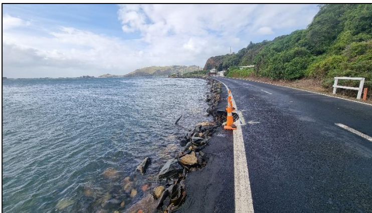
Figure 2 – Otakou Wharf section of Harington Point Road is narrow, being undermined and vulnerable to high tides and sea level rise that will shut off the marae and important businesses unless dealt with as a matter of urgency.
